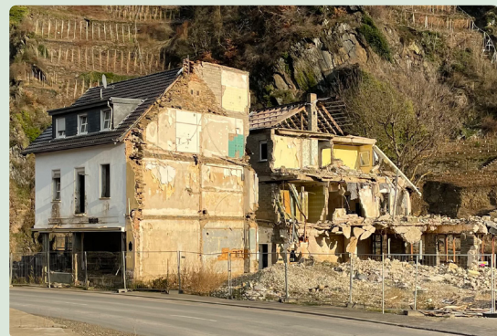
Mayschoss Terraces with flood destruction (January 2024). Source: Valerie Kathawala
